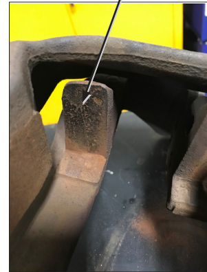
Abutment Surface Rust Removed
